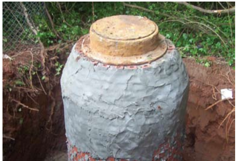
Manhole repair in the City of Atlanta
