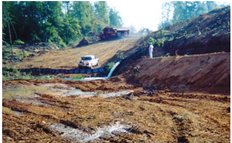
Earth dam improvement under construction
