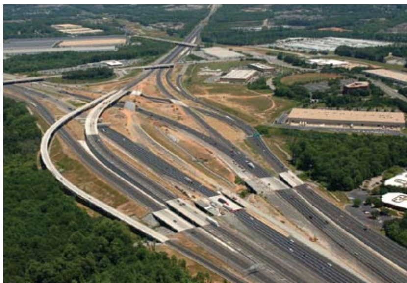
I-85 at SR316 at Interchange
