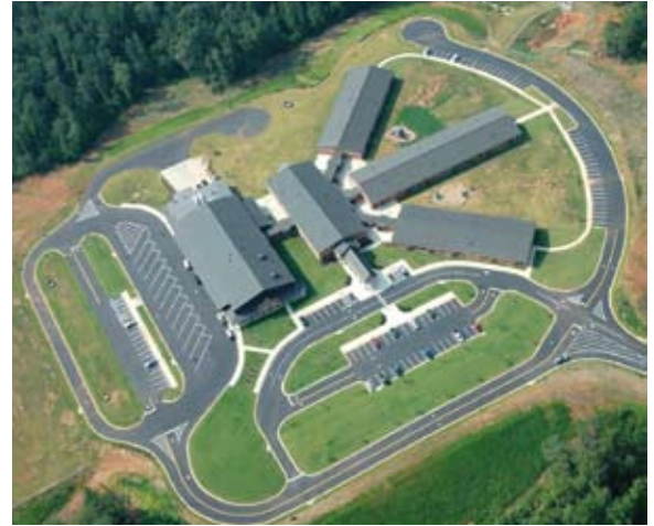
New Elementary School in Troup County
