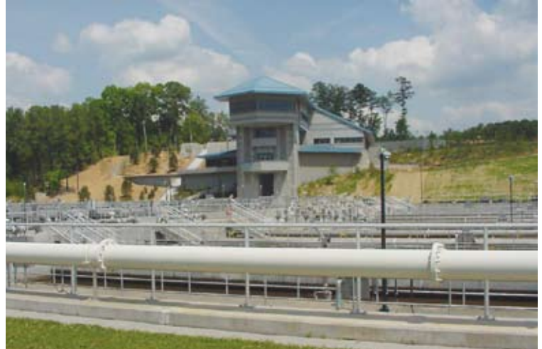
Utoy Creek Water Reclamation Facility in the City of Atlanta
