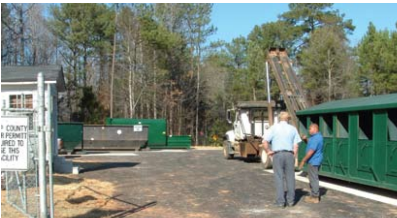
New Solid Waste Convenience Center in Troup County
