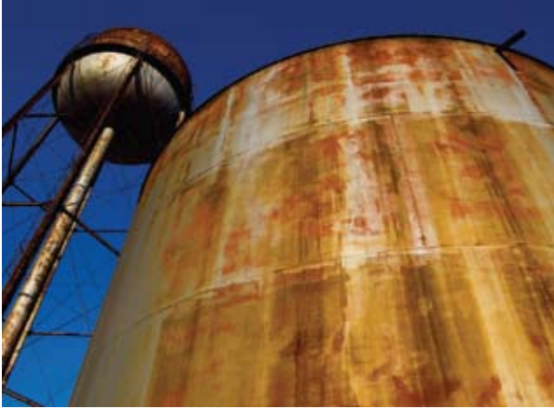
Water Tanks in Rossville, Georgia
